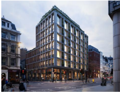
Fleet House, 10 New Bridge Street By Atenor c75,000 sq ft
